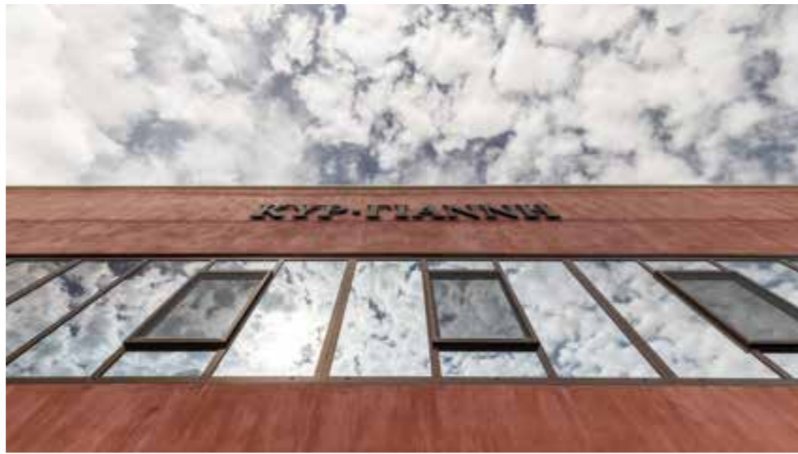
The new Kir-Yianni winery building is a real gem for the region.
